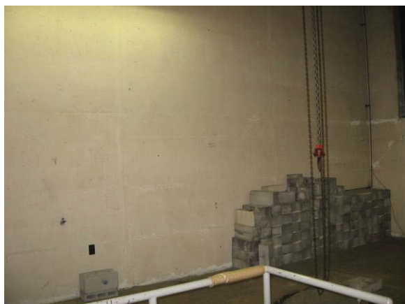
Photograph 2 OTB (Vertical Accelerator Room)
