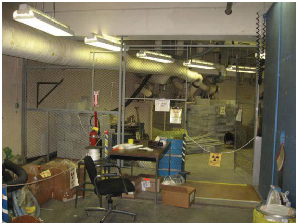
Photograph 59 Main Floor Neutron Level
