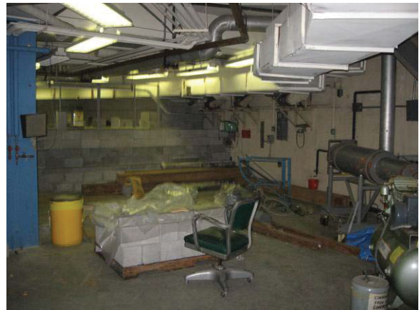
Photograph 62 Main Floor Neutron Level
