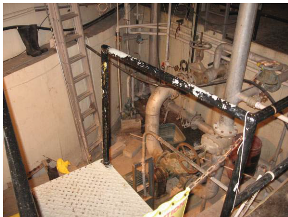
Photograph 30 Room N03 1K Tank Pit
