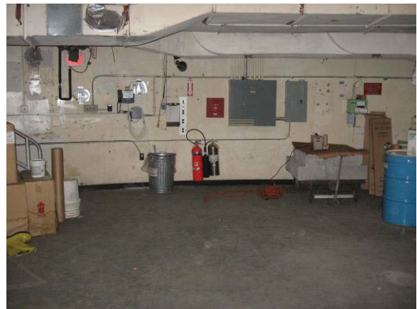
Photograph 63 Main Floor Neutron Level
