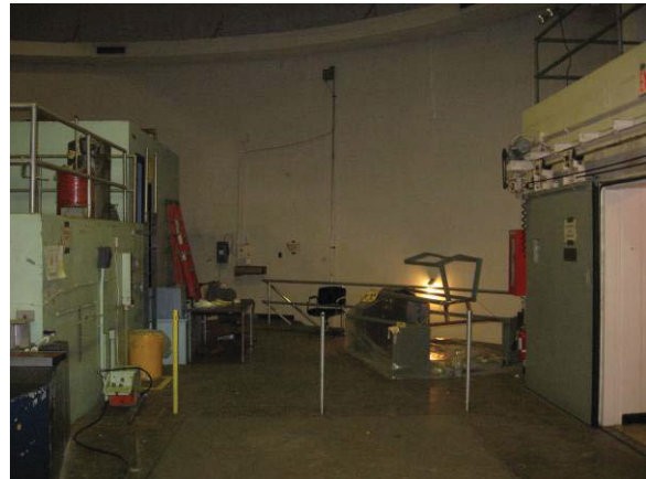
Photograph 42 Main Floor Control Deck
